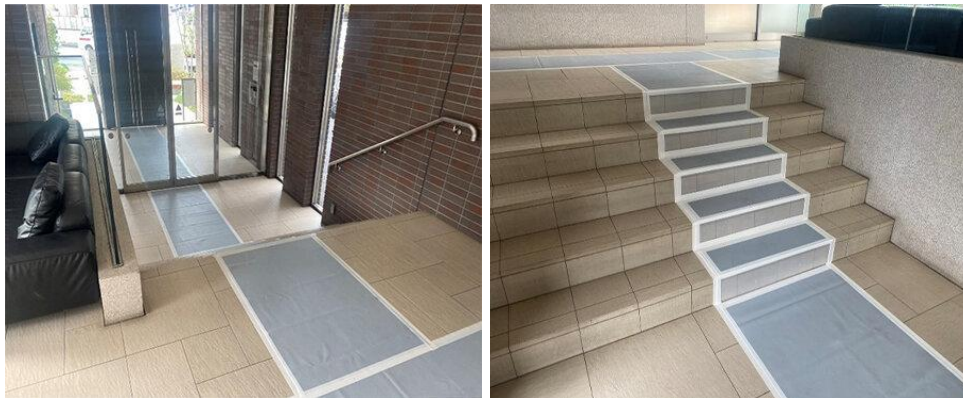
Example of reusable curing sheet use (photo courtesy of Daikyo Anabuki Real Estate)
